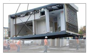
Simultaneously, the object's construction from prefabricates greatly accelerates the work pace. Assembly of a one-floor multi-family building is constructed by a group of 3-5 people and approximately lasts one day. However, the use of segments allows for decreasing the construction costs by 30%.
